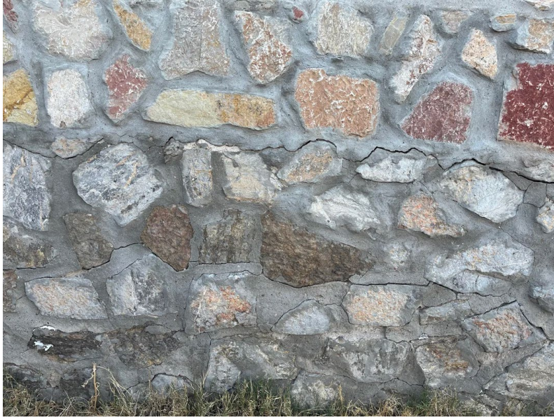
Stone wall with cracks and gaps similar to those noted previously.
