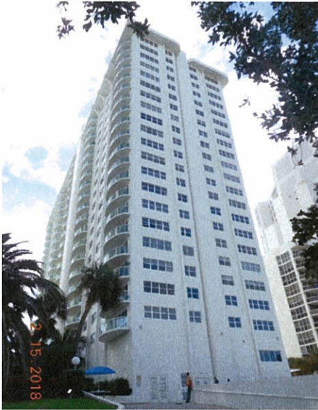
Photo 3.2 South Tower West Elevation
