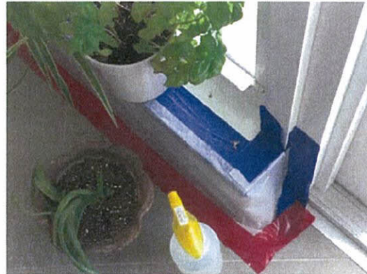
Removed wall panel below balcony window sill due to water intrusion
