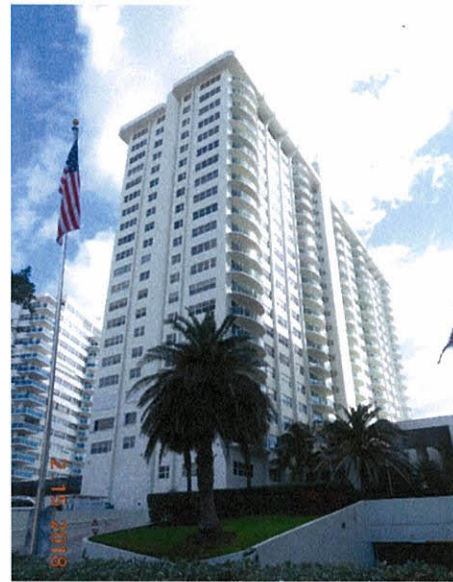
Photo 3.3 North Tower West Elevation
