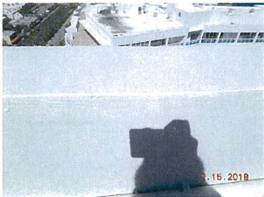
Deteriorated roof deck membrane
