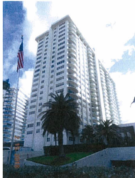
Photo 2.3 North Tower Elevation
