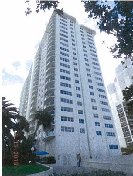
Photo 2.2 South Tower Elevation
